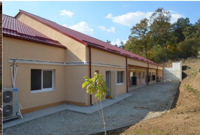
Leamna: After renovation
